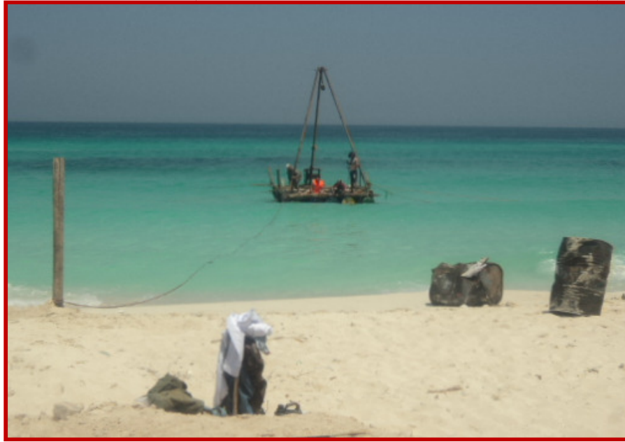
Fig. 4. The bore holes implementation in the site
